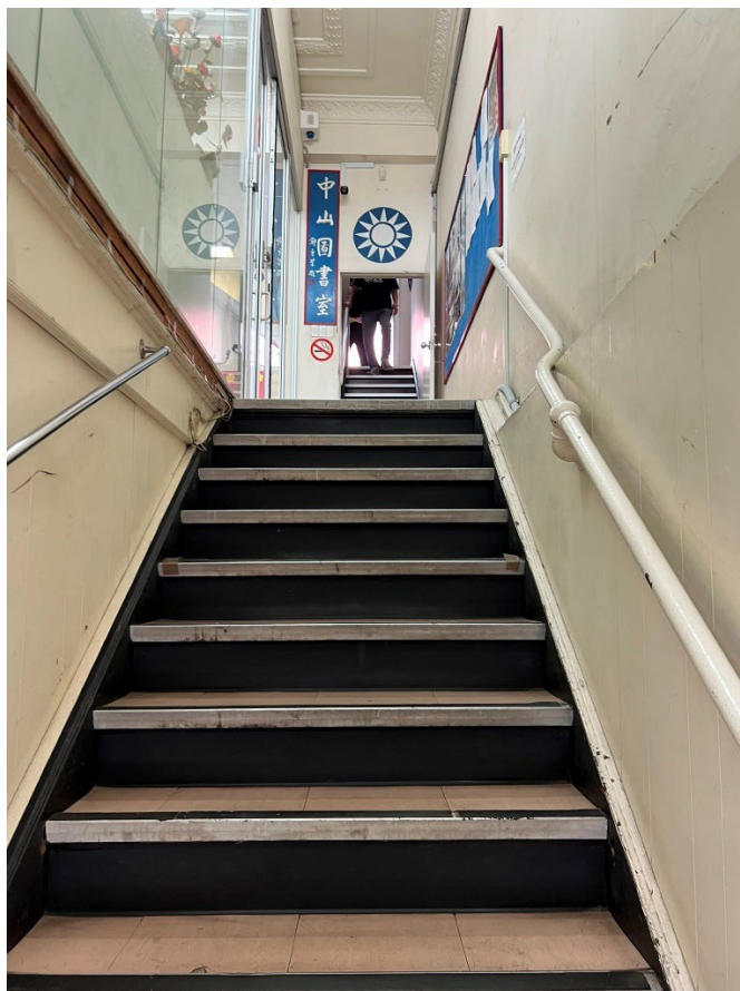
Figure 14 Stairwell to upper floors.
