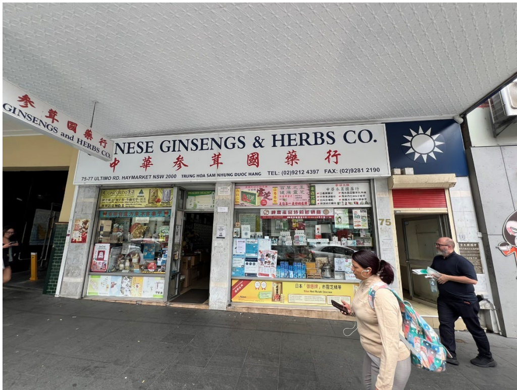
Figure 13 Shop at ground floor of 75-77 Ultimo Road and pressed metal awning.
